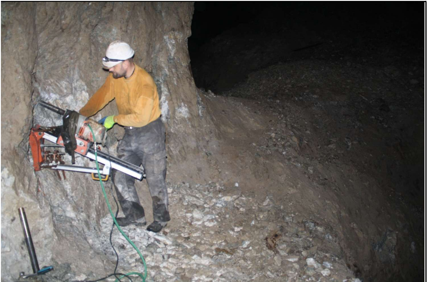
Underground micro-drilling at Schopfer.
